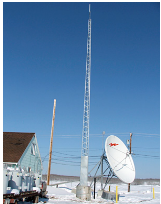
SSI Micro's satellite dishes in the NWT, such as this one in Fort Simpson, are aimed at the Anik-F3 satellite in orbit above the equator. The federal government plans to reveal details of a program to improve Internet access in Northern communities in coming months. - photo courtesy of SSI Micro
